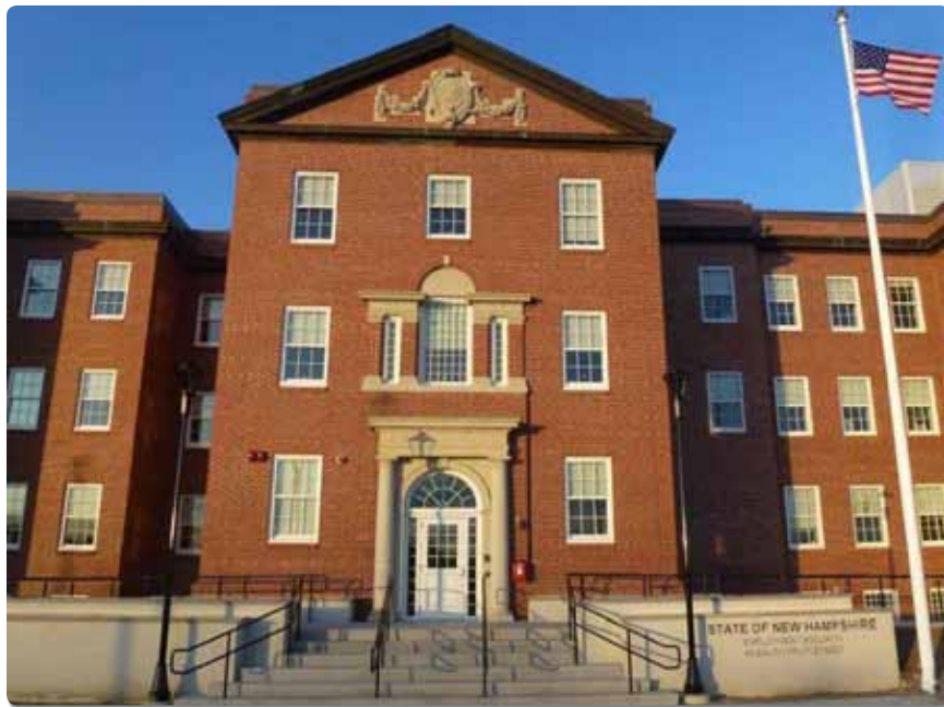
NH Employment Security Administrative Offices Tobey Building, 45 South Fruit Street, Concord, NH
