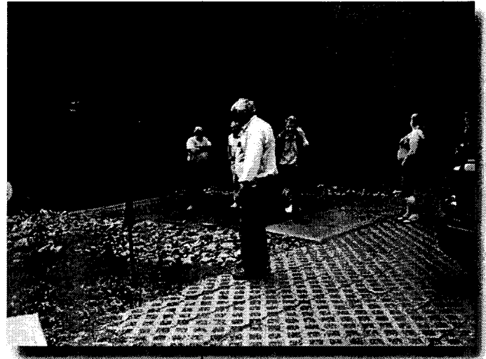
The refurbished boat access site at Hot Hole Pond features precast concrete boat planks and porous concrete pavers.
