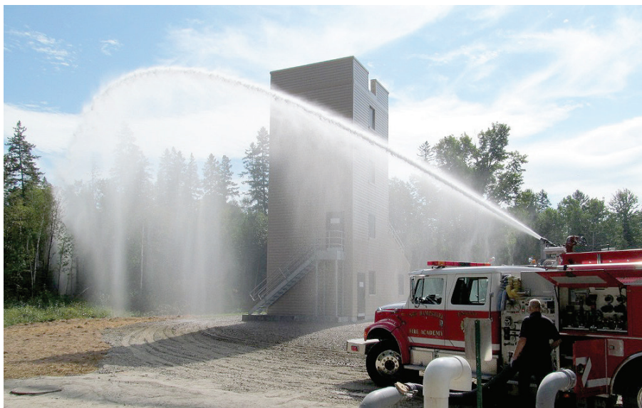
ABOVE: The NH Fire Academy's fire apparatus spraying water onto the fire training structure at the Raymond S. Burton North Country Training Facility in Bethlehem, NH.
