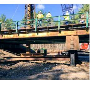
innovative slide-in bridge construction technique. The new substructures will be constructed around the existing bridges and the new superstructures will be constructed on temporary supports adjacent to the roadway while it remains open to traffic. During two separate long-weekend road closures, the existing bridges will be removed and the new superstructures slid into place, completing the new bridges.
