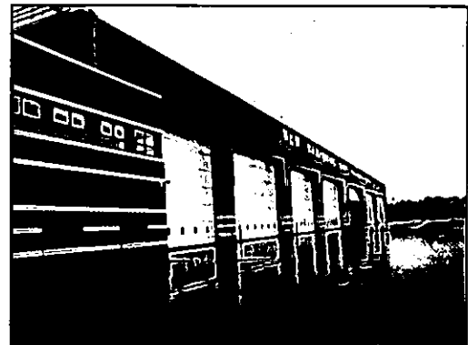
Concord AASF Overhead Doors.
