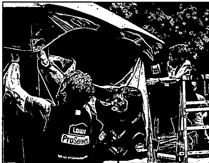
Volunteers from Tilton and Gilford Lowes stores donated and installed a gazebo for NHVH residents.
